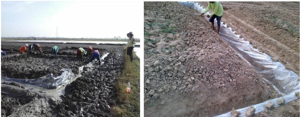
Figure 2.2. Installation of a waterproof sheet around the edges of an experimental plot.
