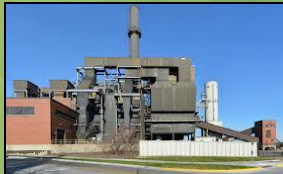
ISU Power Plant
