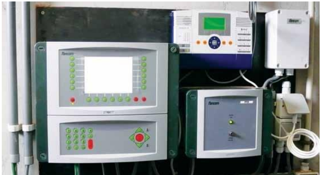
Plate 9: Ventilation computer (left) , battery ventilation system (right under) , Octalarm (right above) .
