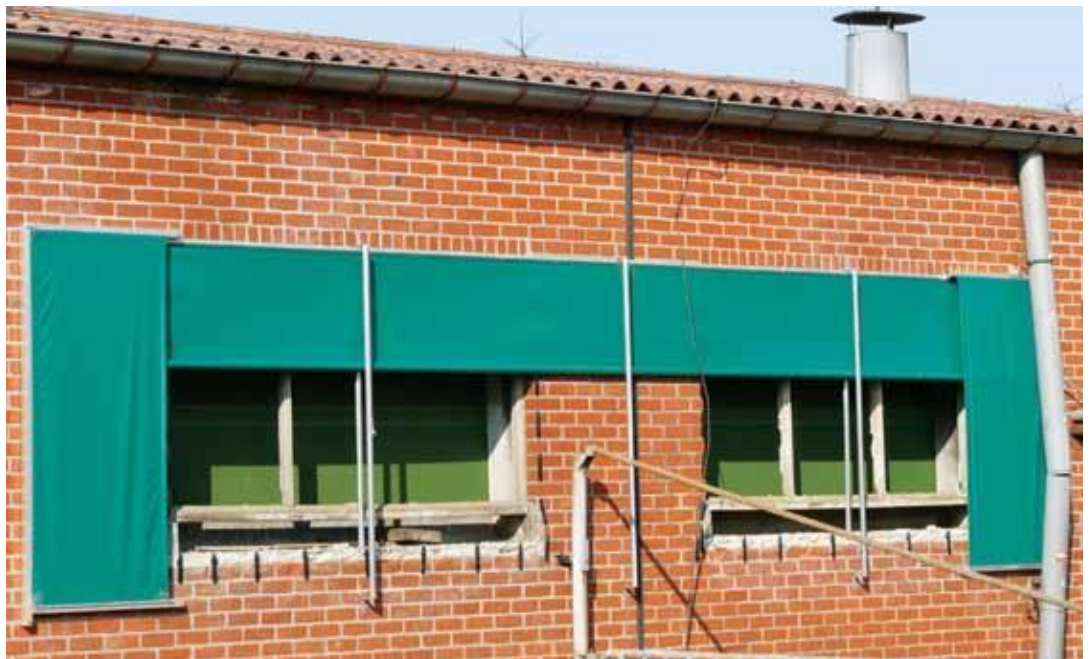
Plate 3: Openings for air inlet, equipped with a fixed wind-breaking net with a porosity of 30% on the inside and an adjustable tarpaulin on the outside.
