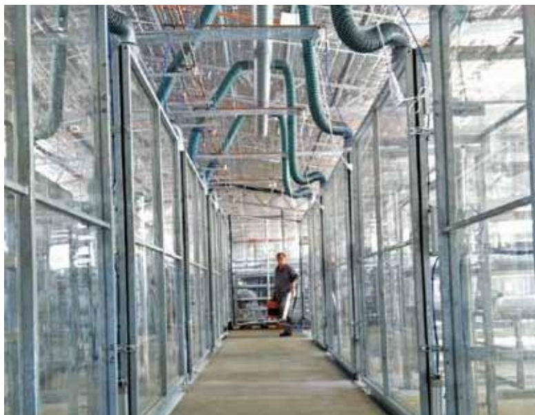
Plate 2: Two rows of five chambers showing aisle between rows, overhead duct and droppers bringing fresh air into each chamber.
