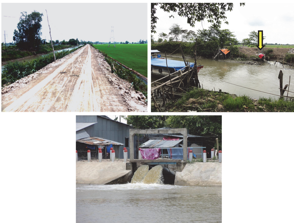
Figure 2.1. A dike system established in An Giang province, Vietnam. (Top left) a bank dividing a canal and fields. (Top right) intake pump for irrigation water to fields. (Bottom) large pumps for drainage to channel.
