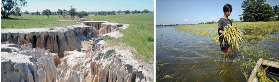
Figure 2: On the left, soil erosion and on the right, flooded rice field .
