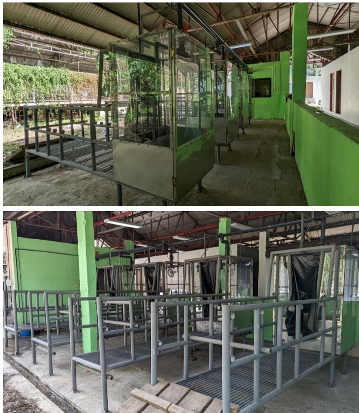
b. The four metabolism stalls equipped with headboxes at the facility
