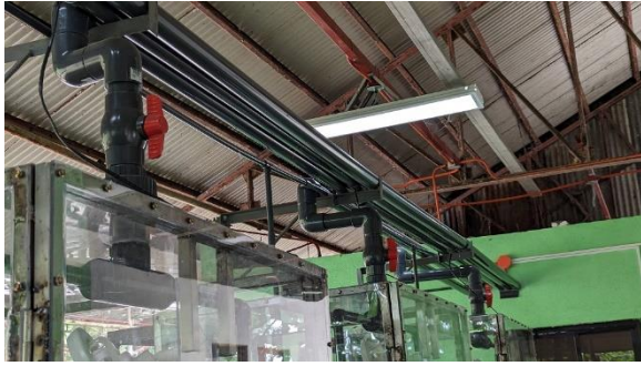
g. Main pipes (2-inch diameter) which direct the air towards the analysis room
