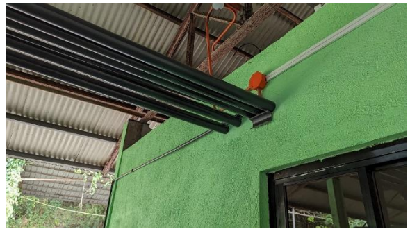
g. Main pipes (2-inch diameter) which direct the air towards the analysis room
