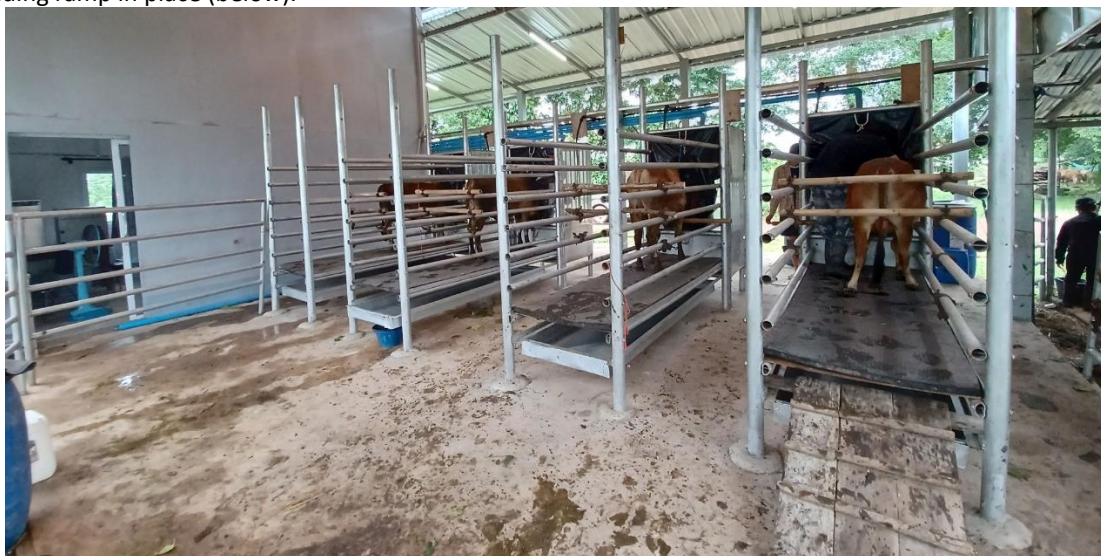
Back of respiratory headbox chambers metabolic crates, showing adjustable back rails and the wooden loading ramp in place (below).
