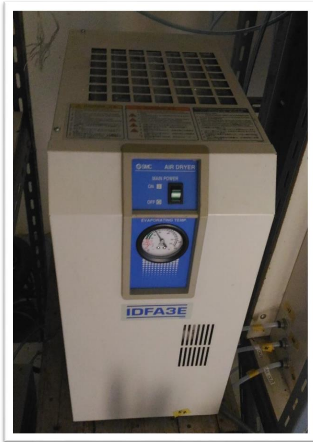
Fig. 9. Air cooling dryer
